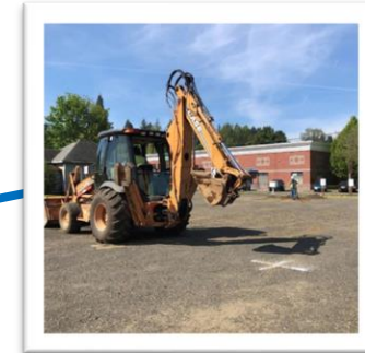
Civic Center parking lot project begins
